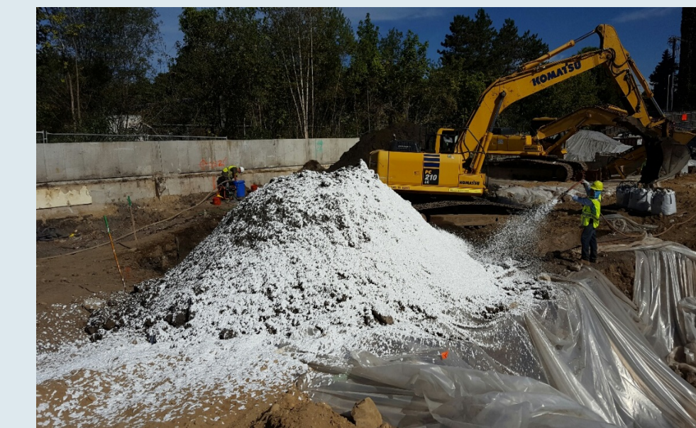
Vapor mitigation activities during soil mixing
